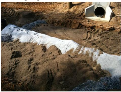
Engineered soil Installed in 1-ft lifts, water in, no compaction
